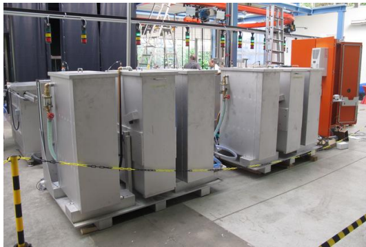
Fig. 11. Doubly installed active carbon filter columns for used wash water recycling
