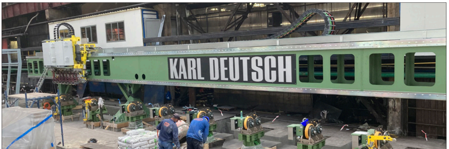
Preparation of grouting activities for the aligned rotary roller stations together with the pipe stopper and the testing bridge
