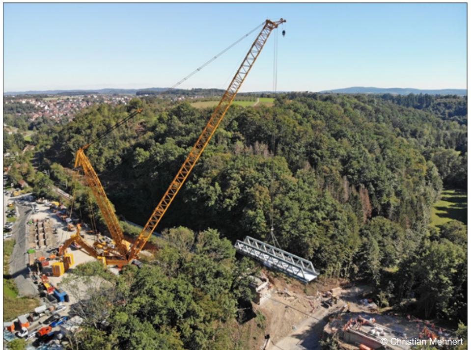
Lifting of the Buchenbach railway bridge with a weight of approx. 190 tonnes
