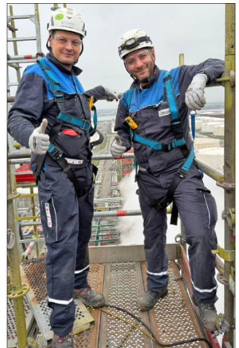
Safety first: preparing for testing at the tank wall
